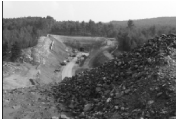
2 short tunnels - these are the mitigation measures for Krusne Hory
